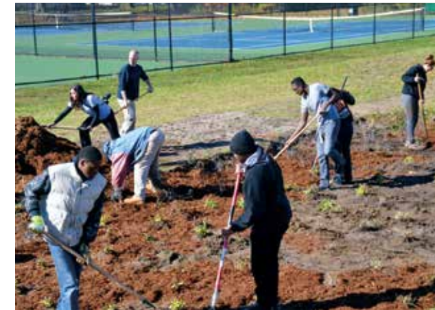
High school students work to install a rain garden as part of a UConn Natural Resources Conservation Academy initiative. (Contributed Photo)
